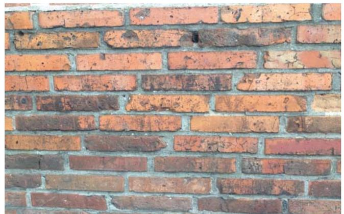
Fig. 11. View of both serviceable and damaged brick wall structure
