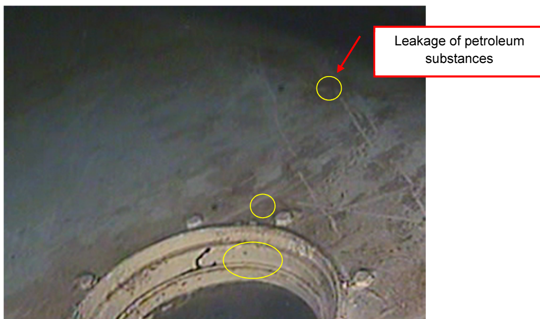
Fig. 8. Leakage of petroleum substances (own studies).
