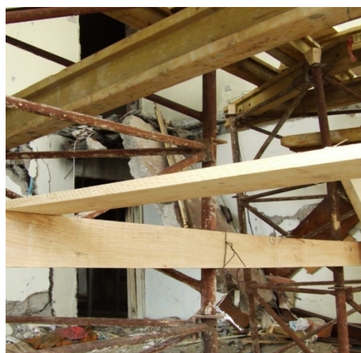
b Failed top slab of the four-storey building in Bacau, 2010 [2]
