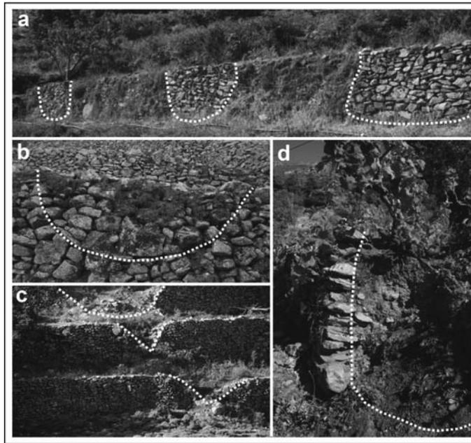
Fig. 9. Exemplary traces of damage done by water and the gravity processes and the results of the repairs done by farmers, observed on plots: a – Vrakades, b and c – Kosikia, d – Prediki
