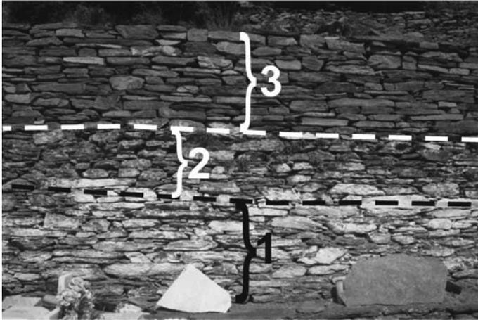
Fig. 7. Stages in the construction of a wall supporting a terrace
