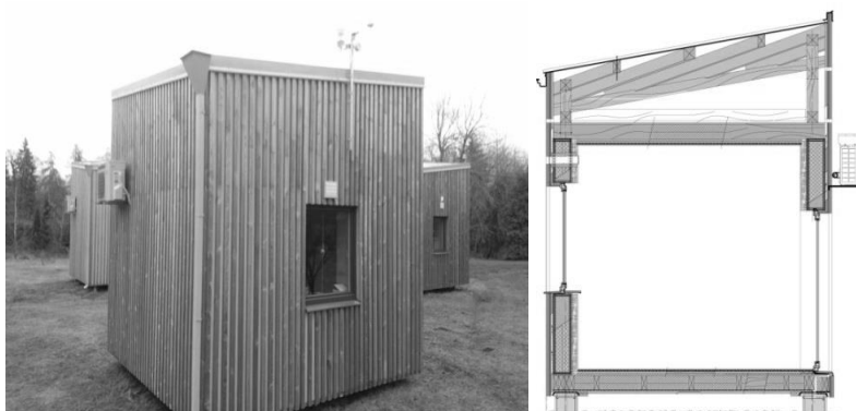
Fig. 1. Experimental test buildings (left) and cross-section of one building with mineral wool filled plywood walls (right).
