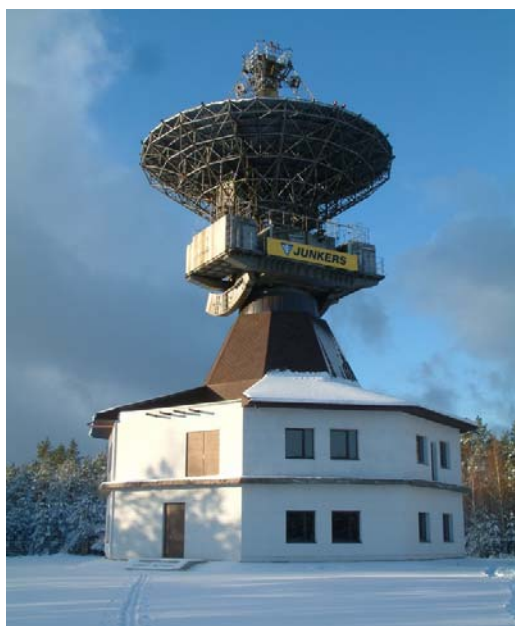
Fig. 1. Radio-telescope RT-16 with a fully steerable antenna.
