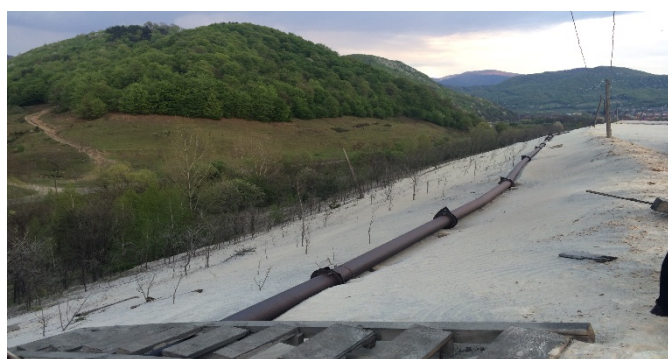
Figure 3: Combating the erosion phenomenon within the decanting pond in Fânațe with the help of forest plantations
