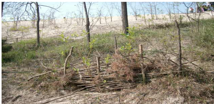
Figure 2: Combating the erosion phenomenon within the decanting pond in Fânațe with the help of silt fences
