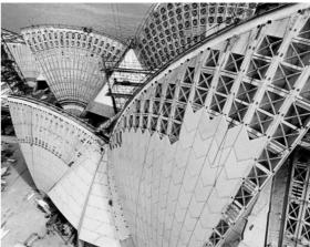
Figure 10. The construction of the gigantic roofs with on-site prefabrication
