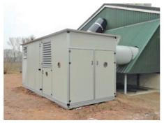
Figure 2. Large central heat recovery heat exchange unit constructed near the barn
