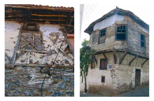
Fig. 6. Himis Technique (Kula) and Bagdadi technique (Bayindir) (right)
