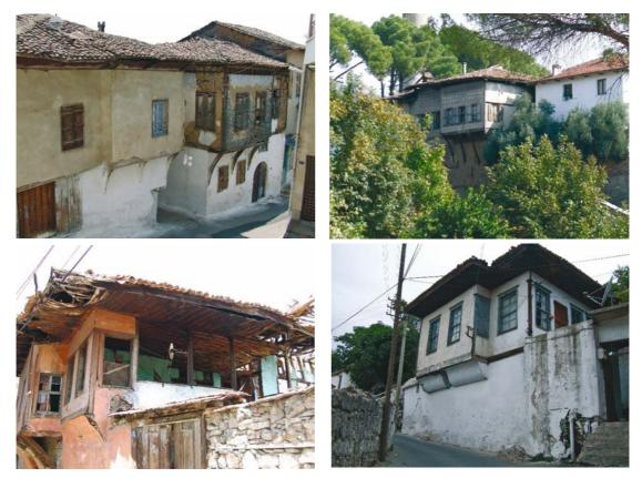
Fig. 9. Different projection types from Bayindir (left up), Kula (Left Down), Birgi (Right Up), Muğla (Right Down)
