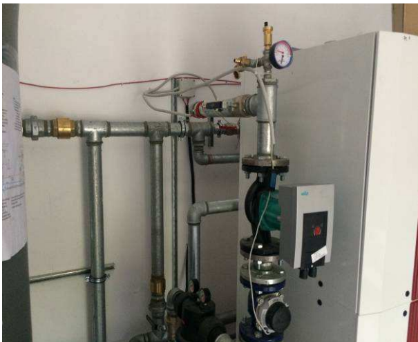
Figure 17. Equipment room flow meters
