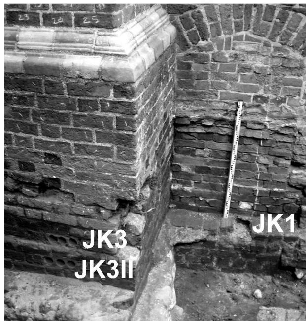
**Fig. 4.** The place of collecting the sample JK3. The discontinuity in the wall construction can be seen. Its presence complicates the geometry of the samples environment that has to be taken into account in estimating the  $\gamma$  component of annual dose.
