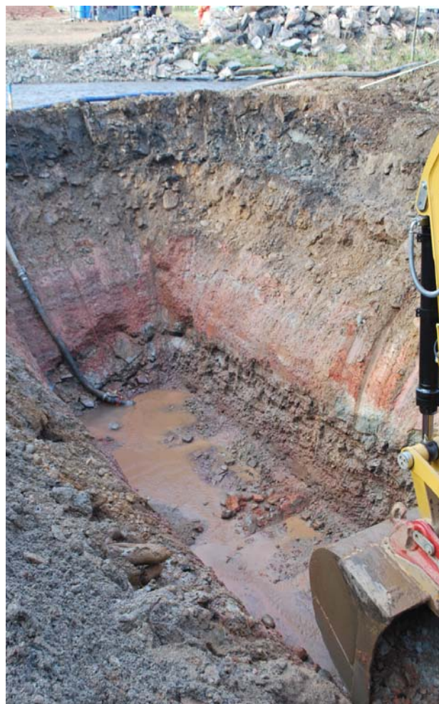
Figure 2. Trench for pipeline near the Czech side of the Svídnice creek. Fine-grained bedded tuffs lie beneath the altered Stephanian clays and Holocene fluvial gravels (NV 389). Photo B. Mlčoch.
