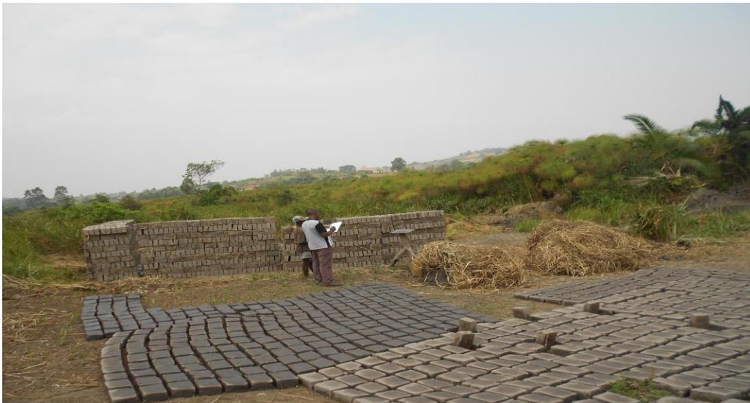
Fig. 3. Bricks that have been made using clay mined from the wetland by one of the members of the local communities in the Central Region, Rusoke, 2013
