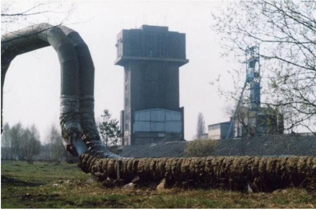
Fig. 3. Winding towers in the closed "Szombierki Coal Mine" in Bytom: "Krystyna" (brick construction) and "Janina" (steel construction) (M. Lamparska)
