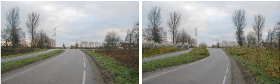
Fig. 7. Dangerous intersection of a road not situated on a dike with a dike road (on the background). Left: In the present situation the road in front leads fluently to the dike road, making the dike invisible. Right: The proposed solution is to accentuate the characteristics of the dike road by planting trees on the dike and a less fluently bend with a sharper slope of the other road (Van Blerck et al., 2009).
