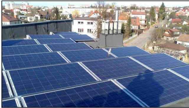
Fig. 10. View of the photovoltaic panels mounted at an angle of  $15^\circ$ , Section 3, on the upper part of the roof [photo: author]
