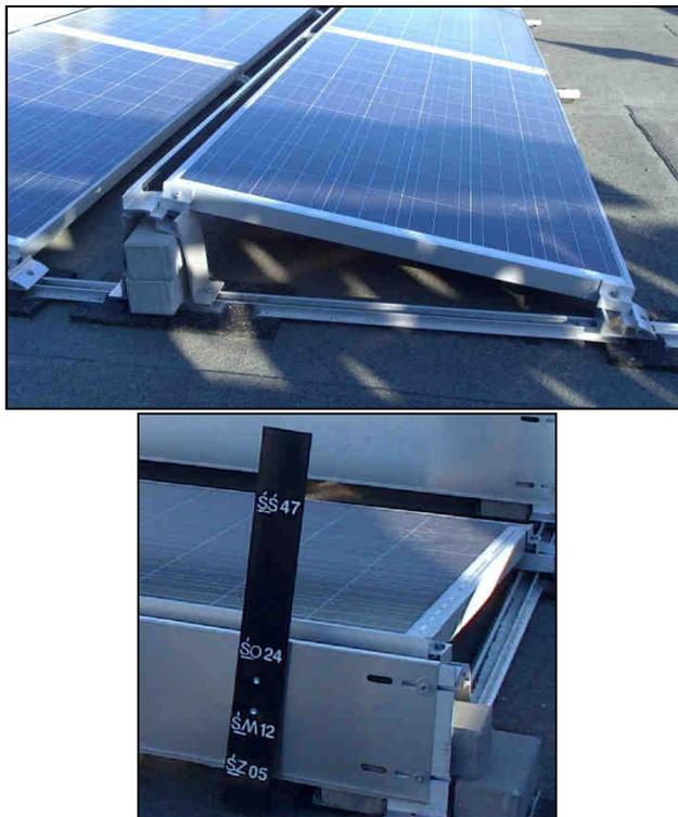
Fig. 7. The setting angle of the photovoltaic panels on the roof of the Ferrox company and safe snow cover indicator [photo: author]
