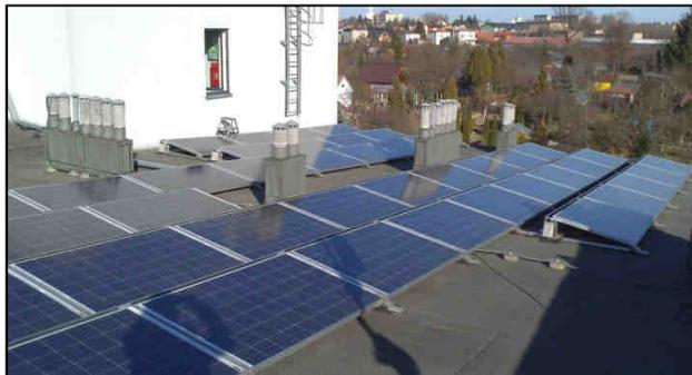
Fig. 9. View of the photovoltaic panels mounted at an angle of  $15^\circ$ , Section 1 and Section 2, on the lower part of the roof [photo: author]
