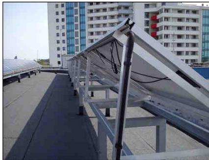
Fig. 6. An exemplary proposed method of photovoltaic panels installation on a supporting structure, for example, the Electrical Technical School building in Bialystok [photo: author]
