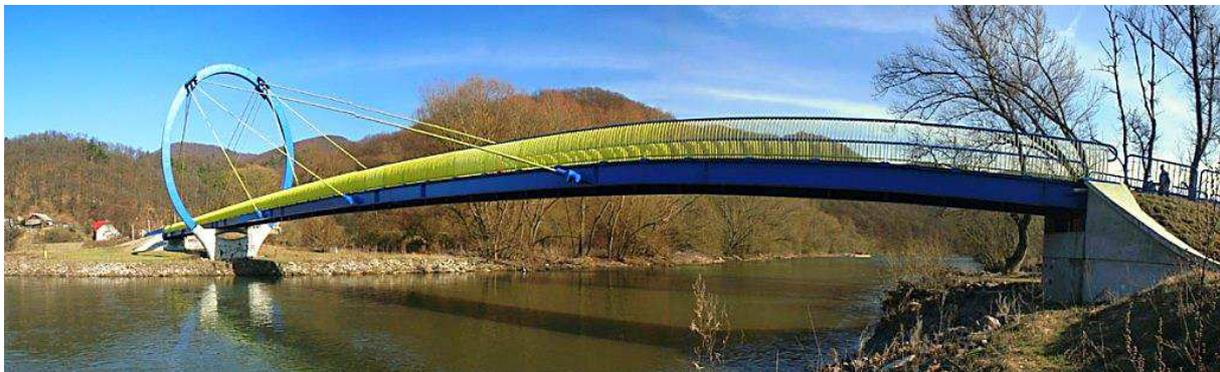
Fig. 1: The steel cable-stayed footbridge in Žarnovica.
