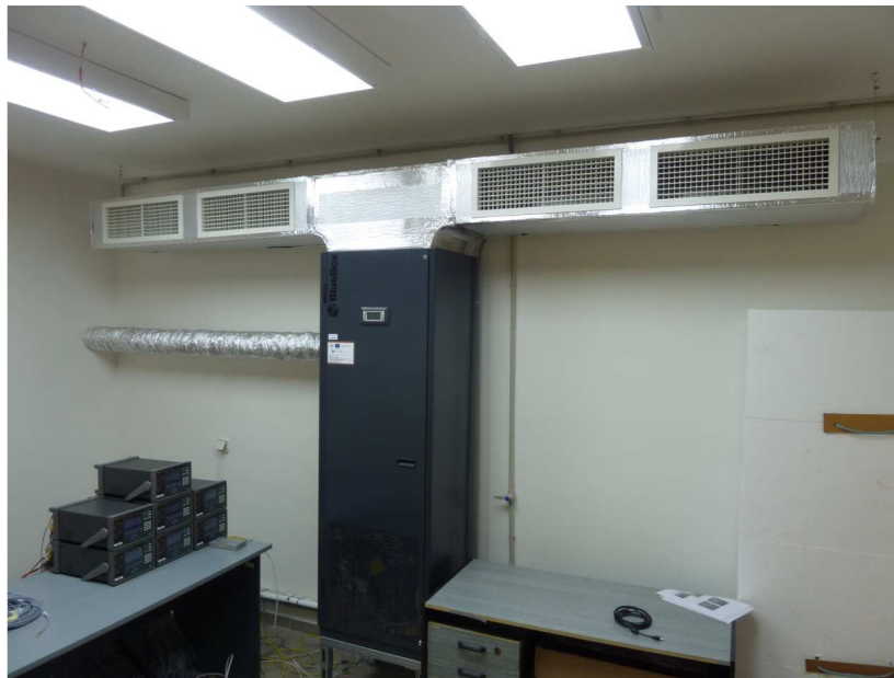
Fig. 8: View at the air-conditioning unit for assignment of indoor environment, multi-channel digital dataloggers and multimeters Hydra III. (placed on the table) [1].
