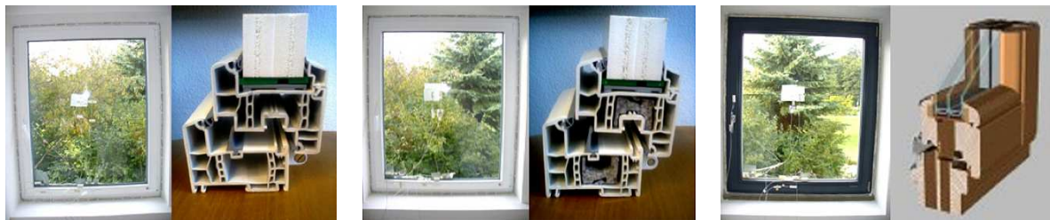
Fig. 1: Interior view of the windows in the building envelope of the pavilion with cuts of frames [9].
