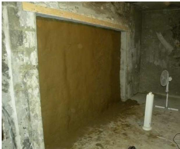
Fig. 5: Drying-out of external clay plaster before measurement. By author.
