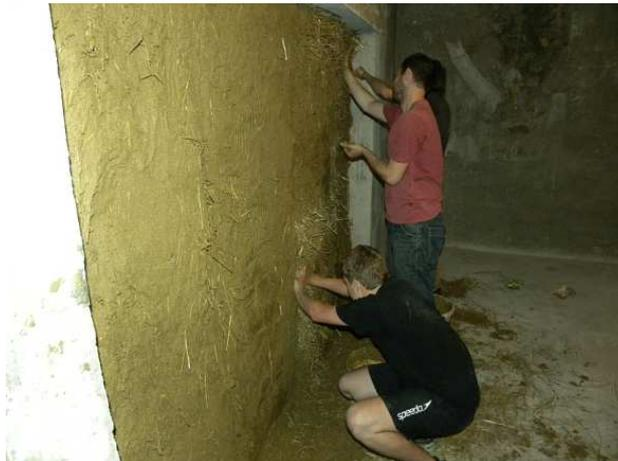
Fig. 4: Application of clay plaster on the straw bale wall surface. By author.
