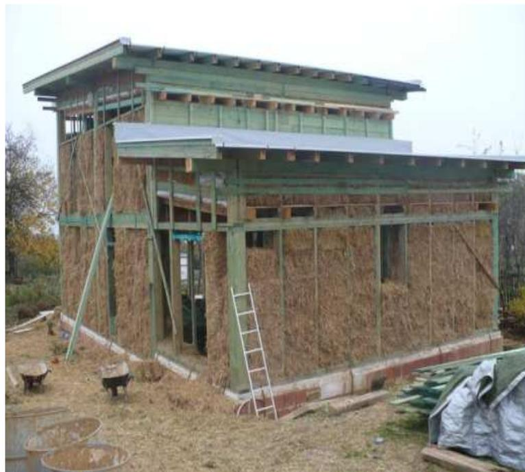
Fig. 2: Example of a straw house in a structural system with a non-load-bearing straw "two by four".
