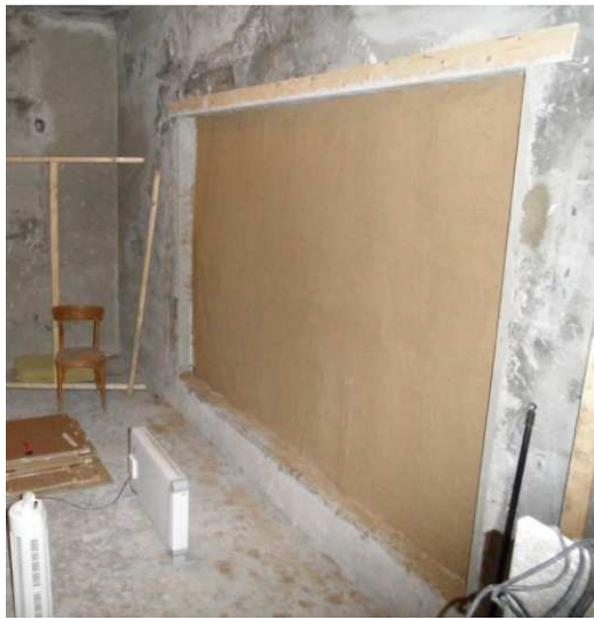
Fig. 9: View of the finished clay plaster on the interior side of the straw wall. By author.
