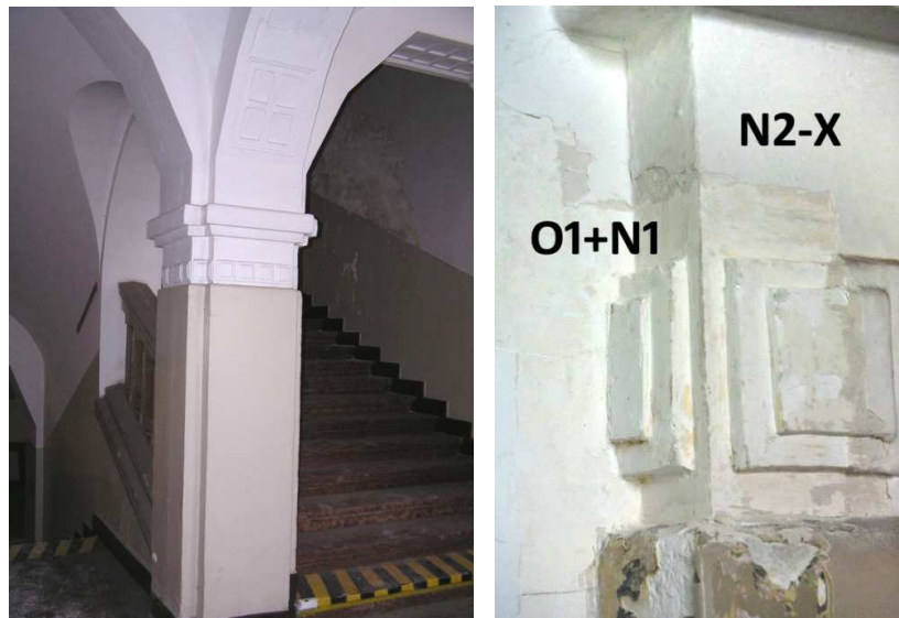
Fig. 2: Gypsum plasterworks at the staircase columns. All the layers are visible:
