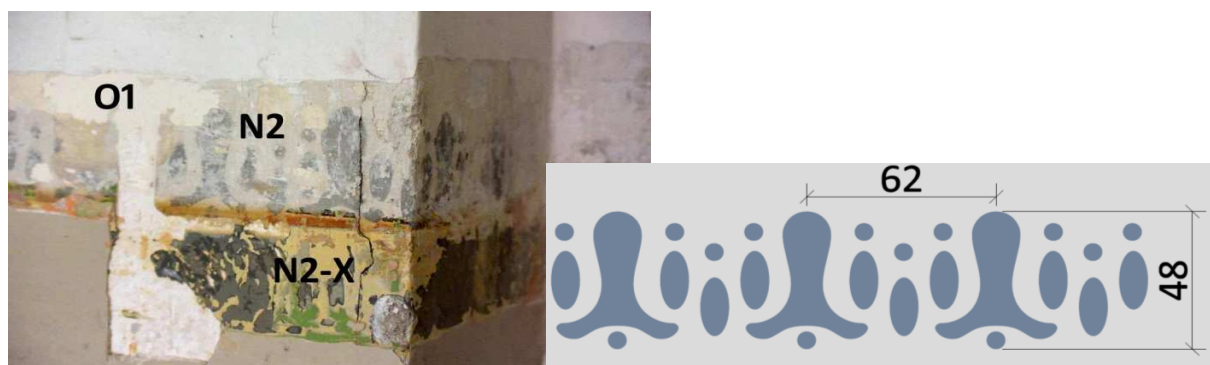
Fig.10: Art nouveau motif, corridor and hall at the 1st to 3rd floor. Dimensions are in mm, based on the in-situ measurement by Bc. Daniela Repaská and Bc. Jozef Smoleň.
