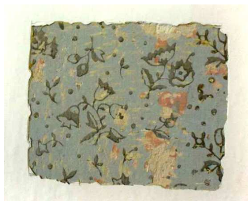
Fig. 3: Example of the modern paint motif (dated circa 1950's), made by patterned paint roller in the Director's apartment at the first floor. Original brown-red hues and ochre layers are visible under the later blue-green-grey paint.
