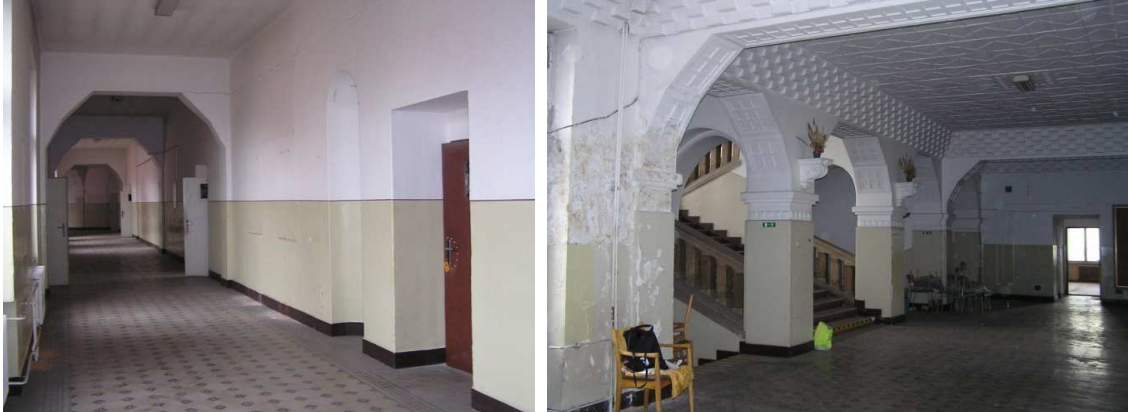
Fig. 4: Present state of corridors and foyer. All final layers are secondary, white paint and beige oil paint. Original ceramic light blue glazed cladding was later painted on, using dark brown oil paint in very thick layers (to be adhesive on ceramic). Reason is unclear, because ceramic tiles and light blue glazing are in a very good condition, maybe to "match overall brownish colour scheme"(?), see Fig. 4. Floor tiles with grey-beige-anthrax carpet theme are also mostly original, but show considerable wear. Band motifs were painted usually just above present brown line dividing white and beige oil paint.
