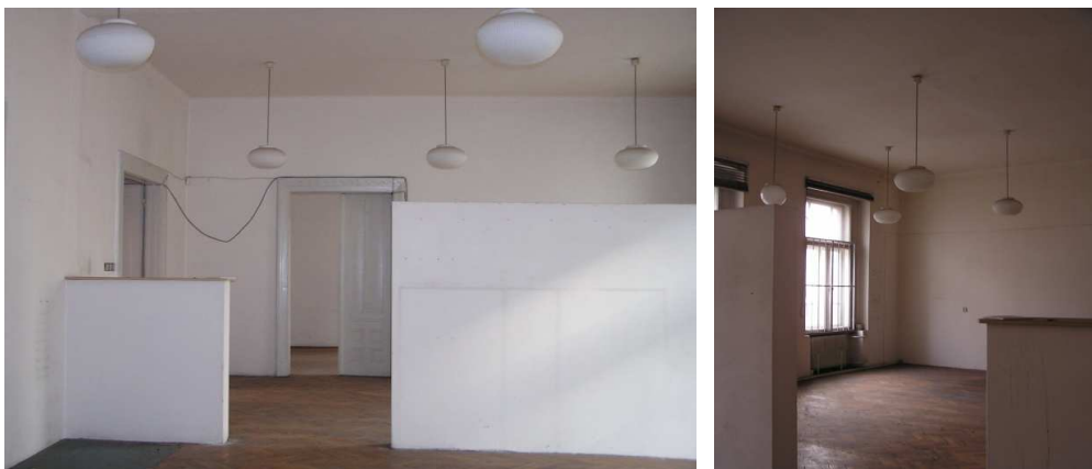
Fig. 5: Present state of the former director's apartment. All final layers are secondary. Note original art nouveau decorated doors (primary glass was replaced by opaque veneer cassettes and painted white). Band motif here encircled the whole rooms at the height of window lintel - motif was so interrupted by window lintel, but ran above doors.
