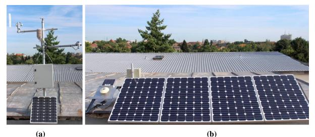
Fig. 1. (a) A photo of the M-UNIT as part of the FORPV toolkit (b) General view of the experimental PV plant PV-L. The equipment is installed on the Solar Platform of the West University of Timisoara.
