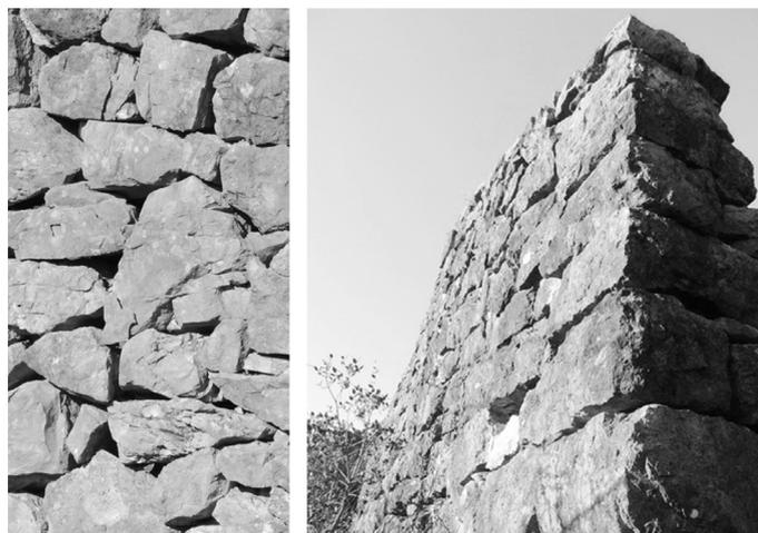
Fig. 15. Stone arrangement—constructing a wall “in dry” [Picture: Irena Rajković].
