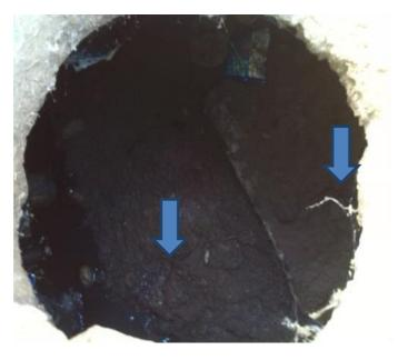
c) Signs of soil erosion and the potential for the total collapse of the VIP.
